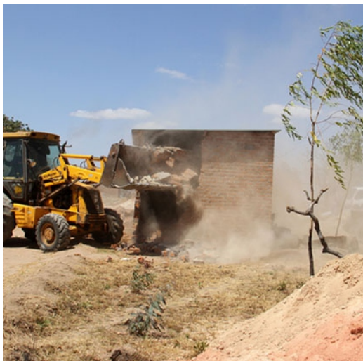
Bulldozer demolishes illegal structures Source - Herald 2021
